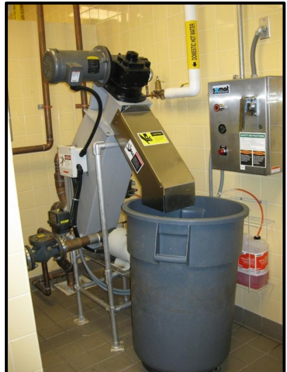
Figure 4. Southside's pulper machine.
